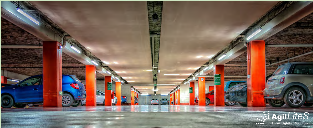
The IoT lighting system can be programmed to adjust luminance according to activity level – creating an on-demand, predictive lighting system.
